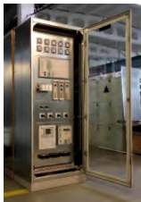
PROTECTION AND TELEMECHANIC CUBICLES IN THE OPU WITH 35-220 KV
