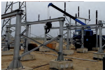
INSTALLATION UNITS FOR ORU WITH 35-220 KV
