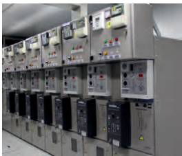
KSO (SINGLE-END SERVICE) CUBICLES OF A REDUCED SIZE WITH ELECTROGAS DISCONNECTORS
