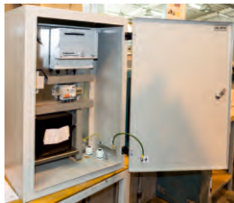
TELEMETRY DATA COLLECTION CUBICLES
