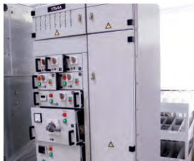
NKU (LOW VOLTAGE DISTRIBUTION SWITCHBOARD) BASED ON A MODULAR SYSTEM
