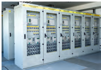
RELAY PROTECTION CUBICLES, SCADA, ALARM AND CONTROL
