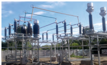
SWITCHES, DISCONNECTORS, GROUNDERS WITH 35-220 KV
