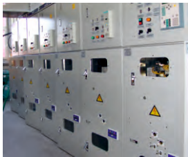
KRU CUBICLES (CUBICLE SWITCHBOARD) WITH SWITCH IN CASSETTE UP TO 3150A/40KA
